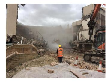
Phase 4 – Demolition The 4 storey, concrete framed building was demolished using remote techniques with various excavators.
