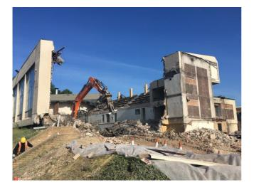
Phase 5 – Crushing Crushing was then undertaken onsite, producing aggregate to 6F2.
